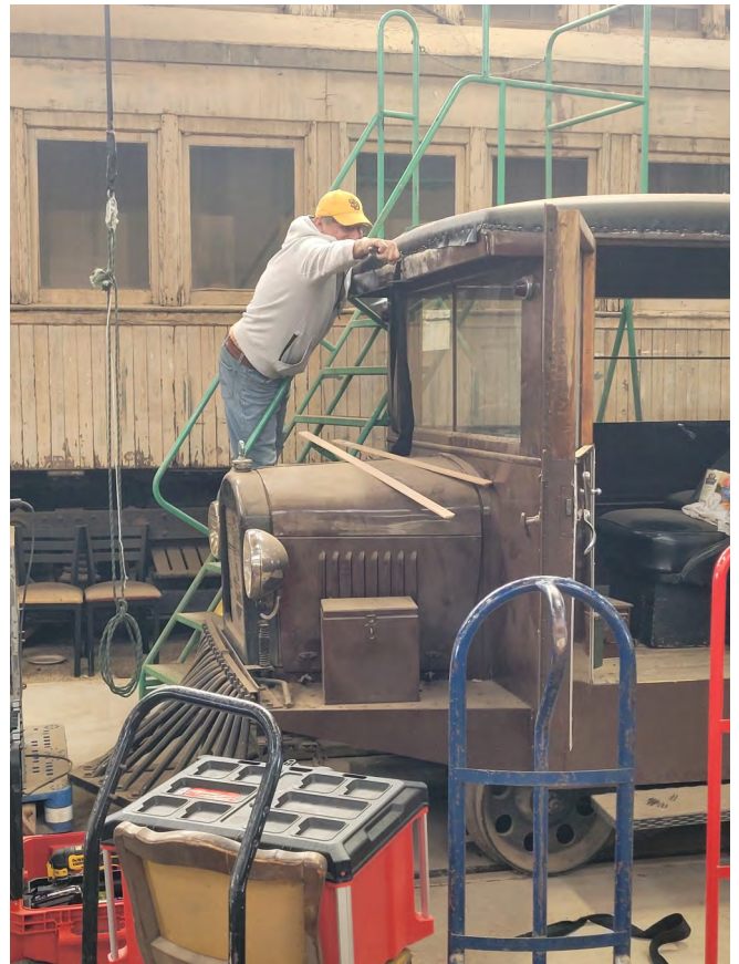
Frank Najera continues to install a new roof on the 1932 Santa Maria railbus. https://www.psrn.org/trains/passenger/smv-9/
