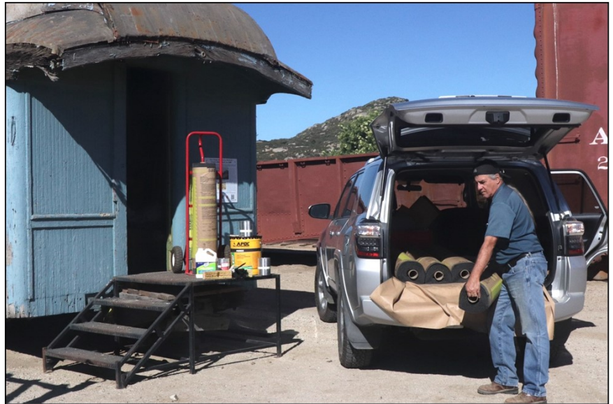
Richard Finch unloading roofing materials for car #240.
