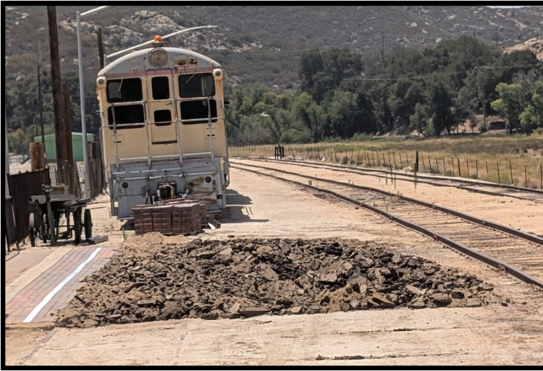
Removal of old, broken asphalt was the first effort required to allow for the placement of bricks.
